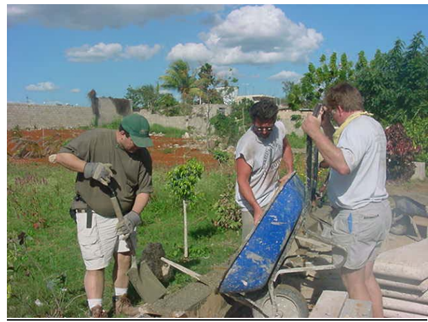
Pouring cement on a construction project.
